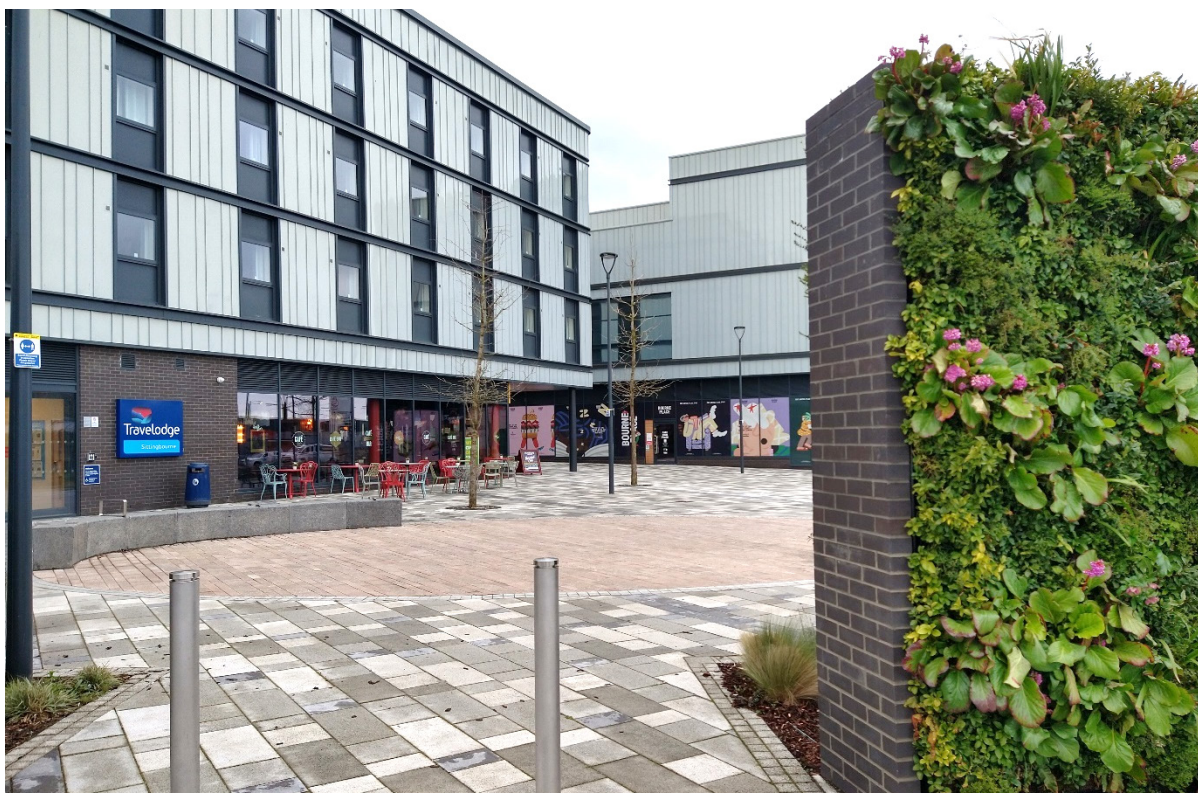
Bourne Place, part of the new connection between the railway station and the High Street
